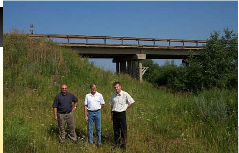
Dr. Harik, Simpson and Nikolai Bogoyavlensky, bridge engineer with the Perm Road Committee, at the Tiskovka Bridge
