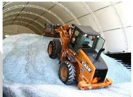
The Woodford County Maintenance Facility recently received a new salt storage hangar.
