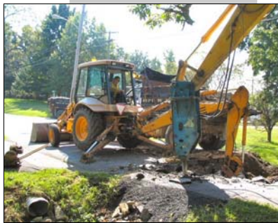
Clark County Maintenance Personnel replaces a cross drain on KY 1927 (Colby Road) between KY 1958 ( Winchester By-Pass) and KY 627 (Boonesboro Rd).
