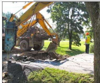
Clark County Maintenance Personnel replaces a cross drain on KY 1927 (Colby Road) between KY 1958 ( Winchester By-Pass) and KY 627 (Boonesboro Rd).
